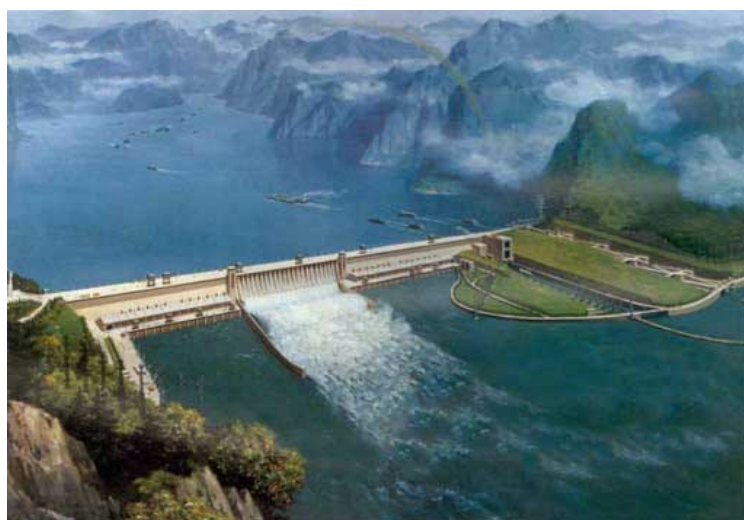
Figure 9 Hydropower station in China
