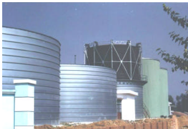
Figure 10 Biogas project of food process factory in China
