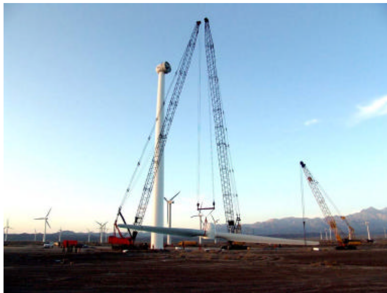
Figure 3 Installation of domestic 1.2MW wind turbine in 2005
